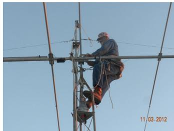
Bert securing repaired yagi boom
